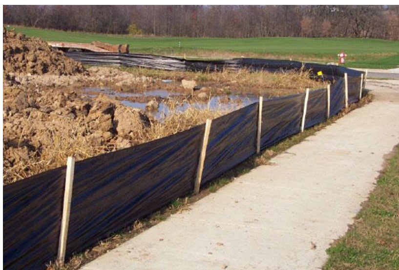
Typical silt fence to be employed.
